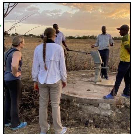
The Team discovered the pump at Nyamahanga was out-of-service (drilled in 2010).
